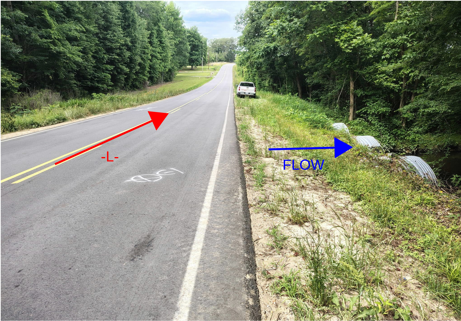
LOOKING NORTH AT SOUTH END OF THE PROPOSED CULVERT LOCATION
